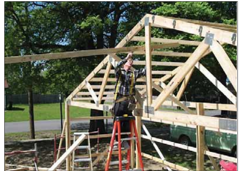
Stephen Rhodes works on the Wardrobe addition in Hayti.
