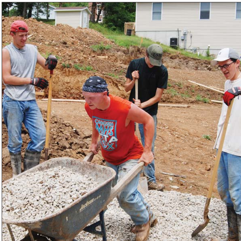
Trent Kiefer pushes a wheel barrow of rock to a foundation.
